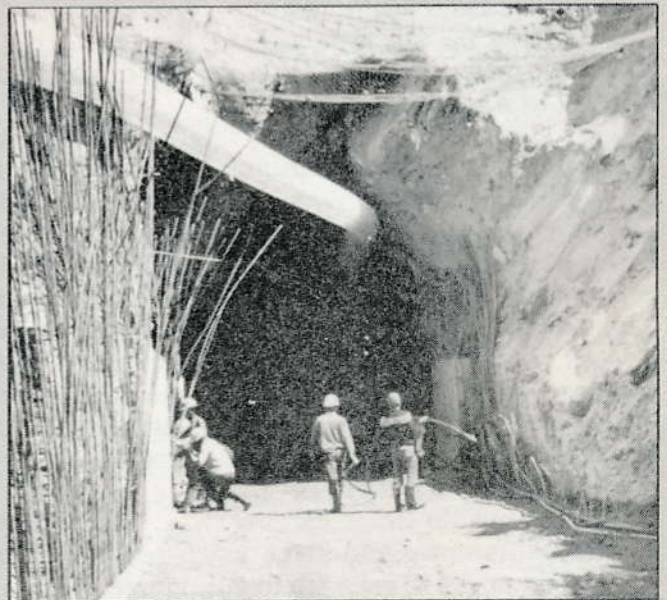
Tunneling works in Khimti ■
